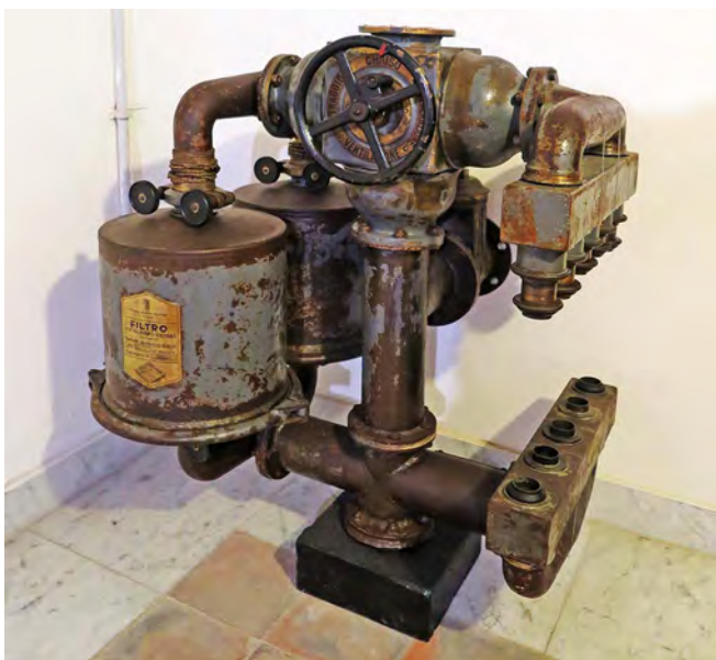
Mussolini's second air-raid shelter beneath the main house. This is the air filtration unit and pump and contains activated charcoal
